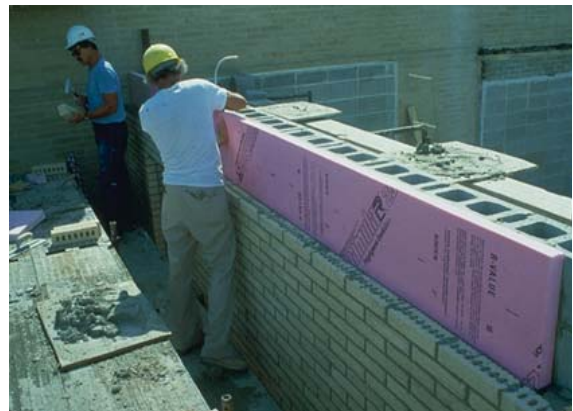
Figure 5: Masonry Cavity Wall
