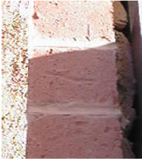
Figure 6: Mortar Bridging
