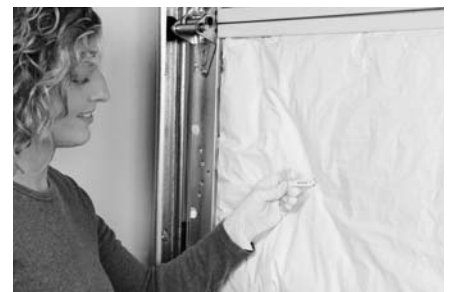
Install Retention Clips
