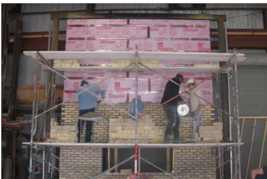
Figure 3: Test wall under construction
