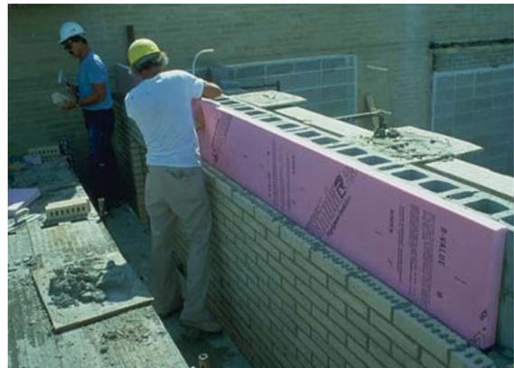
Water that enters the air space cavity migrates downward. Along the way it may encounter imperfections in construction like mortar bridges (Figure 6) that conduct it across the air space cavity to the face of the insulation and possibly to the inner masonry wythe.
